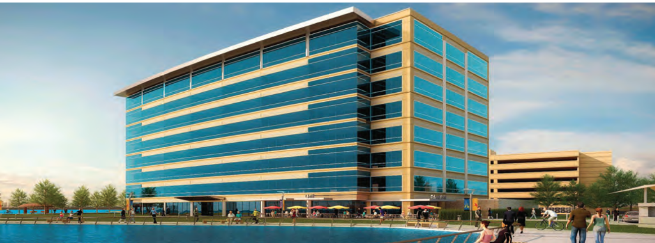
ONE HUGHES LANDING, HOUSTON, TX
